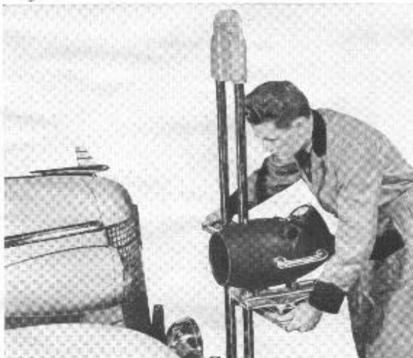
1. The Robot is first centered with the car and then located in front of headlight.
