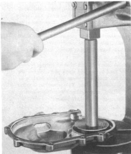
FIGURE 14—Installation of Timing Chain Cover Seal
