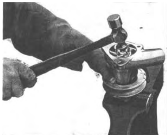
Figure 515—Peening Shaft
