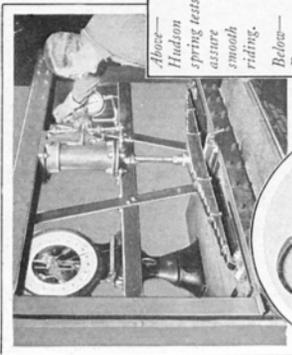
Above—Hudson spring tests assure smooth riding. Below—Every connecting rod Brinnell-tested for hardness.
